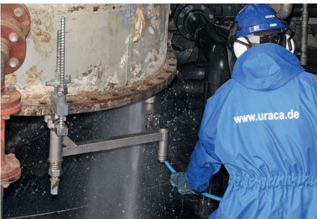
Heat exchanger cleaning with retaining device
